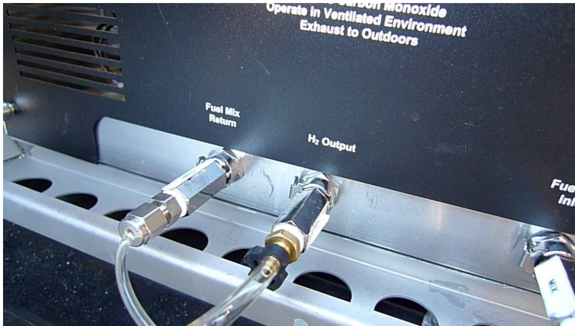
Hydrogen output from reformer.
