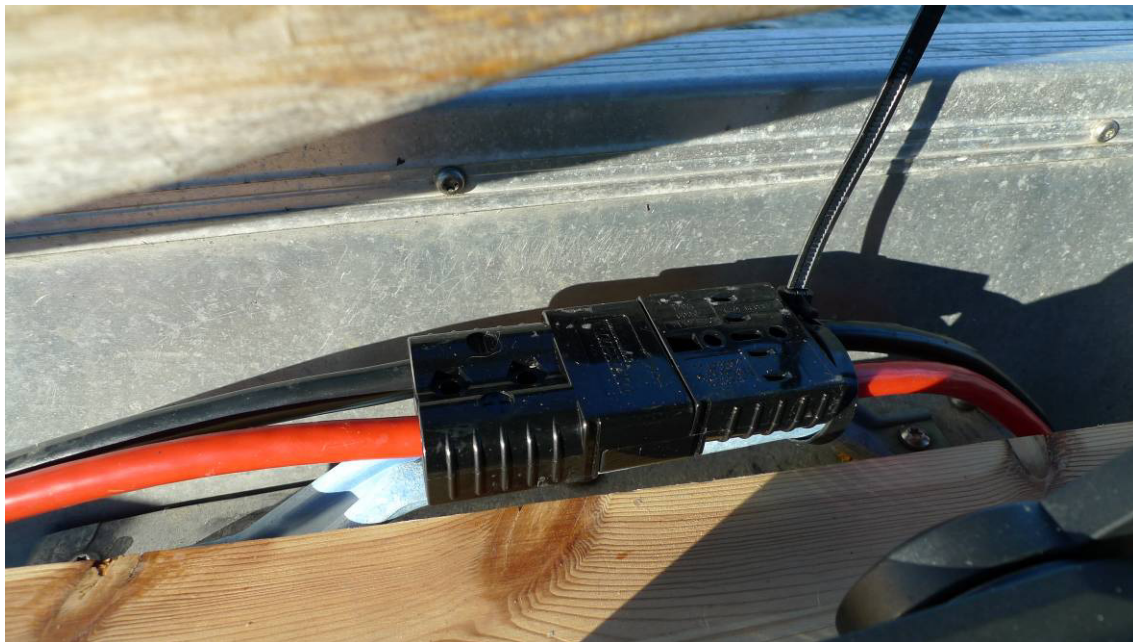
Electric cable to motor.
