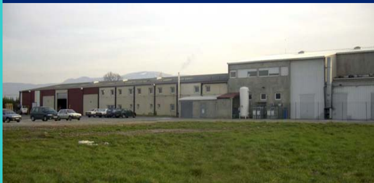
Plant at Romans - Drôme
